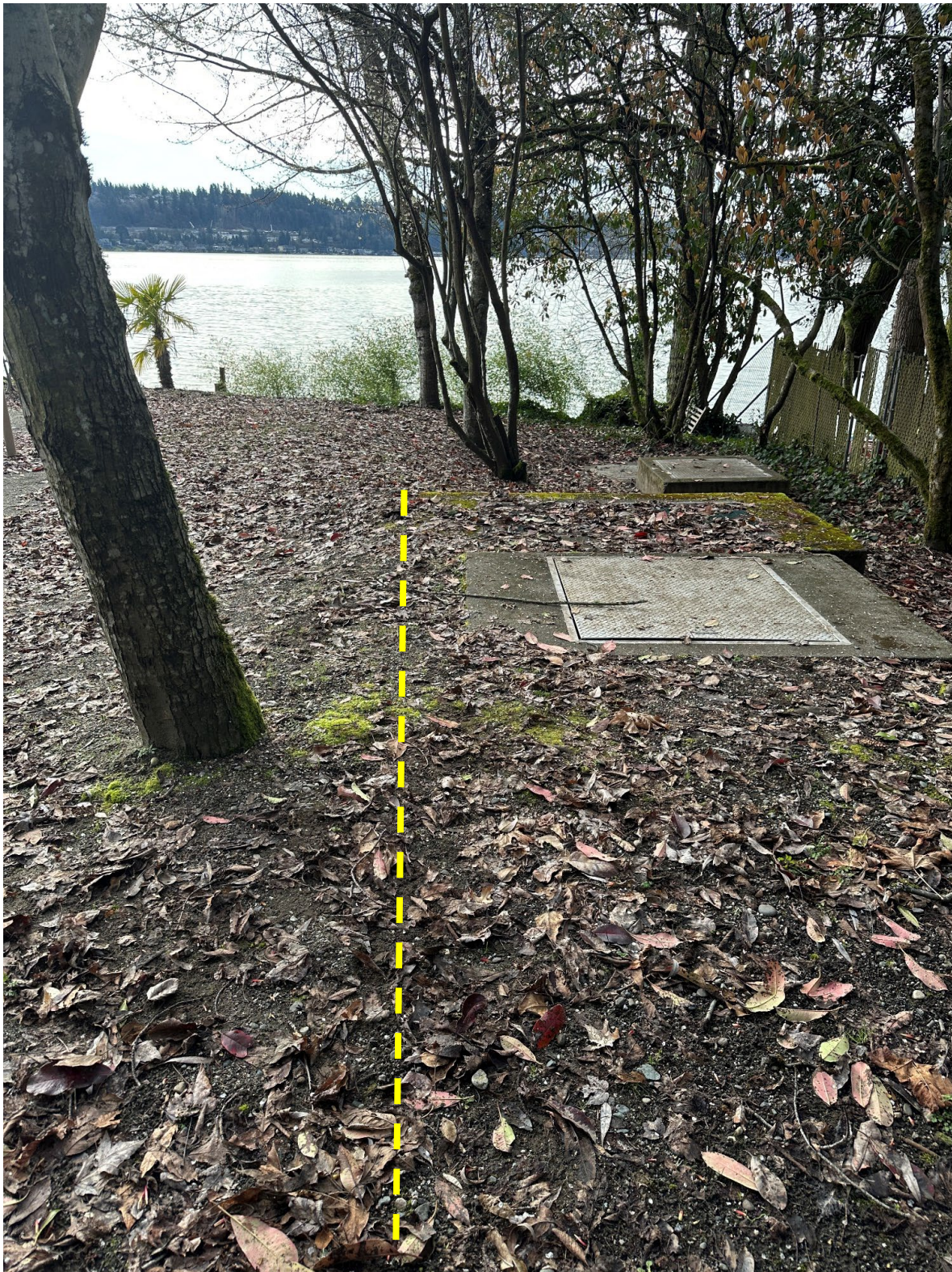
Photo 2. The edge of the concrete lid was less than 3 feet from the trunk of the red maple. The yellow dashed line is the approximate edge of the lid. A shallow layer of soil covered the lid. The viewer is looking southeast.
